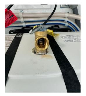
(if the pressure relief value is ever leaking or dribbling water it can be re-seated. Remove the water pressure by letting water out of the line with the van unplugged.
